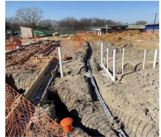
Ongoing Installation of Building Electrical Conduit.
