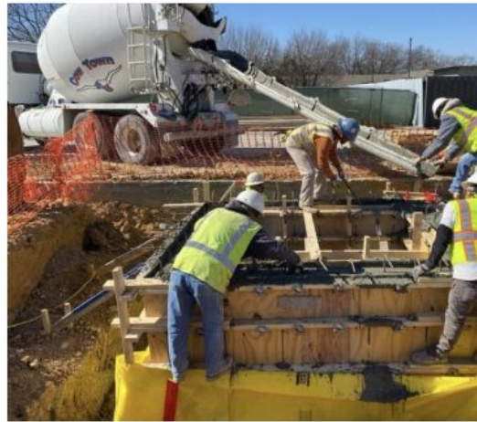
Completion of Elevator Pit Pour.
