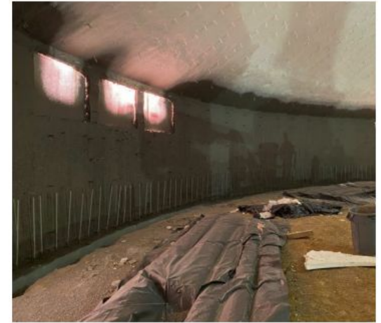
¾ in Spacer Layer for Dome Walls Complete.
