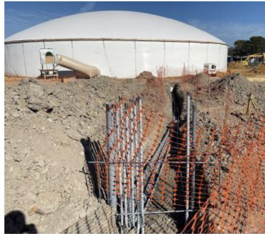
Ongoing Installation of Building Electrical Conduit.
