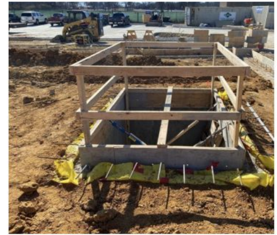
Completion of Elevator Pit Pour.
