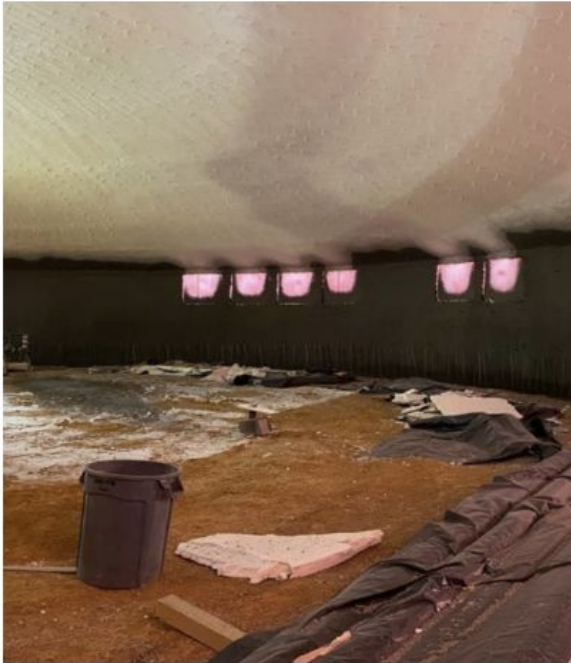
¾ in Spacer Layer for Dome Walls Complete.
