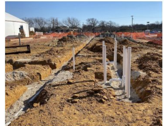
Ongoing Installation of Underground Building Plumbing.
