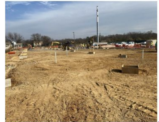
Ongoing Backfill, Grading, and Formwork in Preparation for Slab on Grade Pour.
