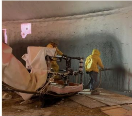
Ongoing Application of the ¾ in Spacer Layer in the Dome.
