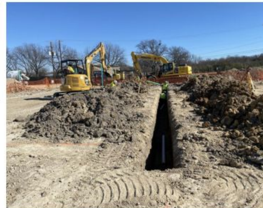
Ongoing Installation of Underground Building Plumbing.
